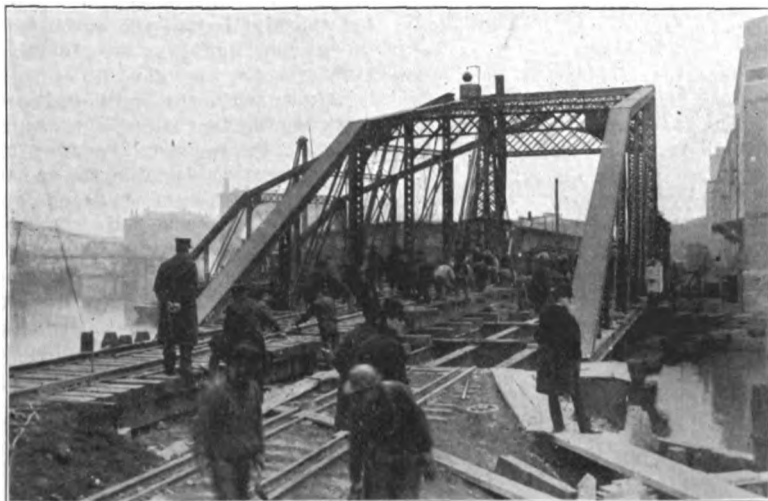
FIG. 6—NORTH END CLOSED AND TRACK BEING LAID, 2:40 P. M.
