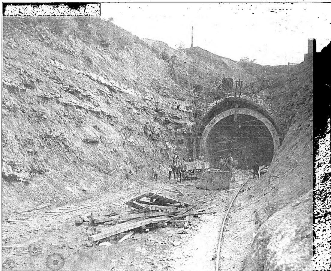
East Portal, Greentree Tunnel, showing Approach and Brick Lining.
